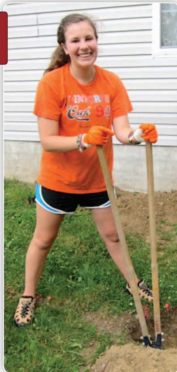
Conistonians dig in ... working to build a ramp with Habitat for Humanity
